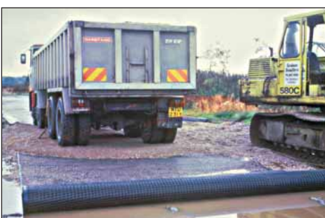
Figure 1: Simple practical demonstration of the benefits of Tensor biaxial geogrid.
