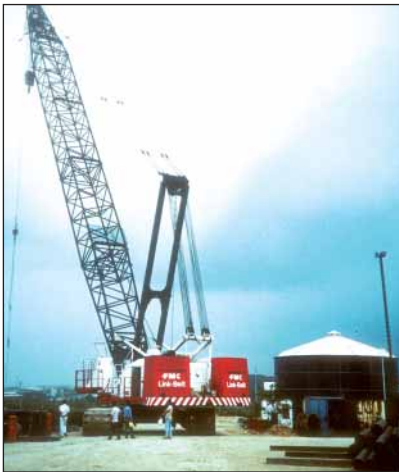
Figure 2a: Crane used in trial.
