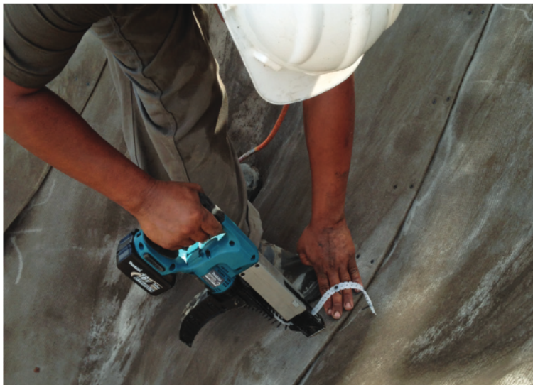
Joints were screwed every 200mm with a double row of screws
