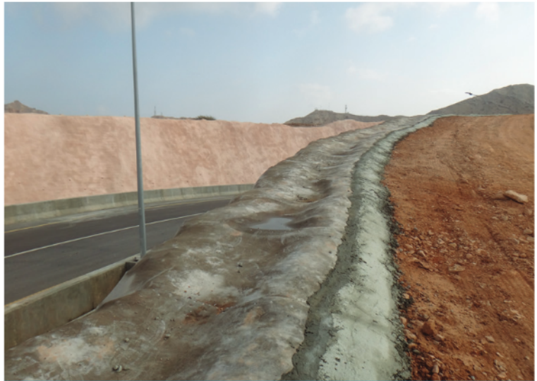
Anchor trench at the crest of the slope
