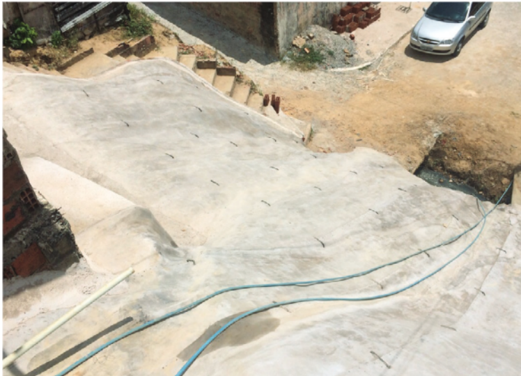
The finished painted slope
