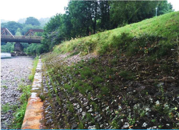
The rip-rap embankment prior to installation
