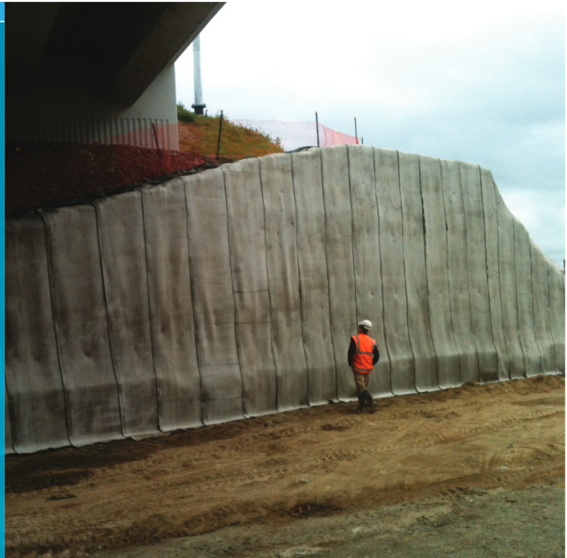
Completed section of slope lined with CC5
