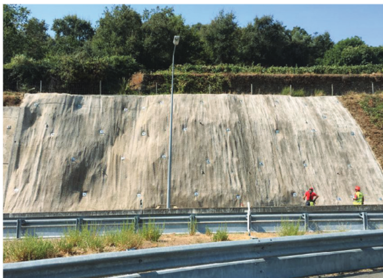
The completed installation of slope
