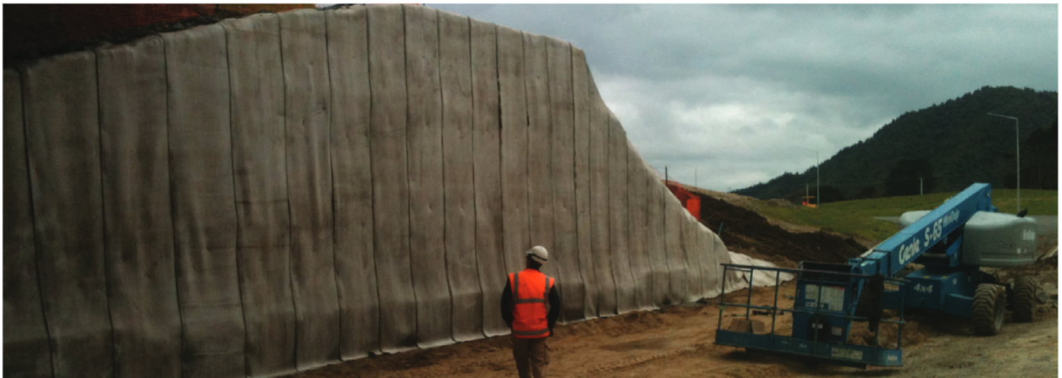
Completed section of abutment
