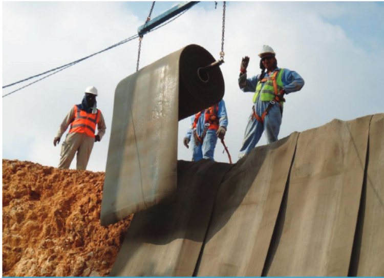
CC being lifted into position
