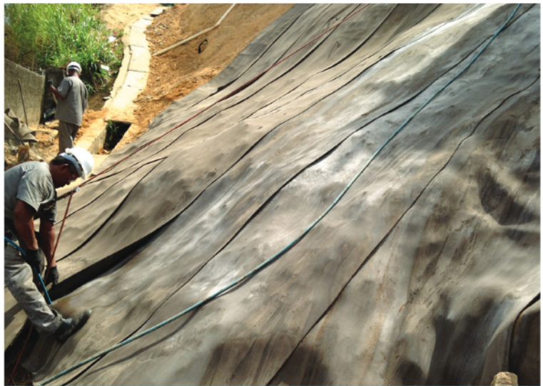
Hydrating under the overlap
