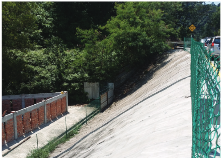
The completed project 18 months after installation
