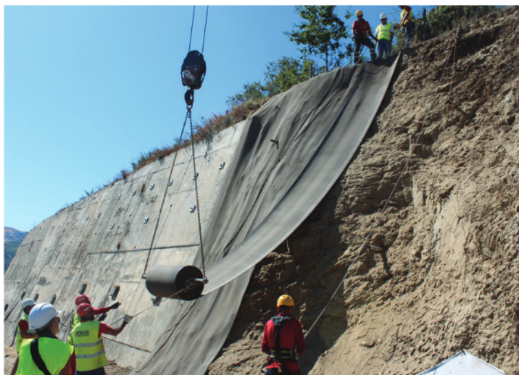
Vegetation and any large rocks were removed, prior to installation
