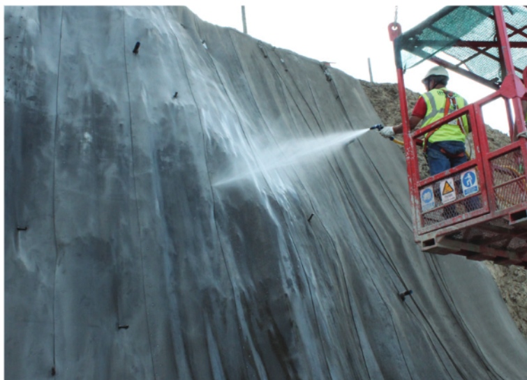
Hydration was achieved using two 1000ltr water tanks with spray nozzle
