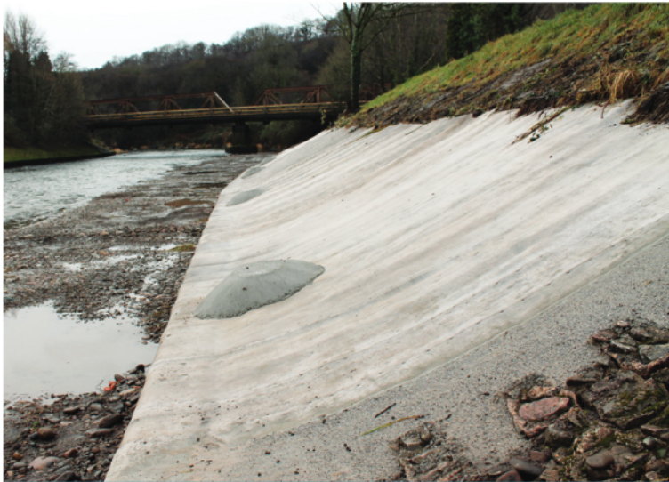
Grouted termination to rip-rap
