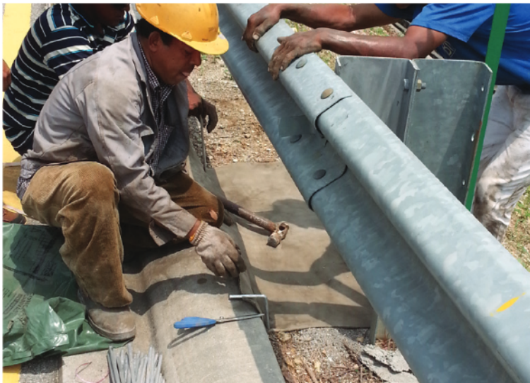
Fixing at the crest with ground pegs
