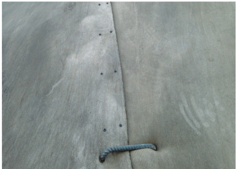
Pegs were inserted through every overlap at 2m intervals
