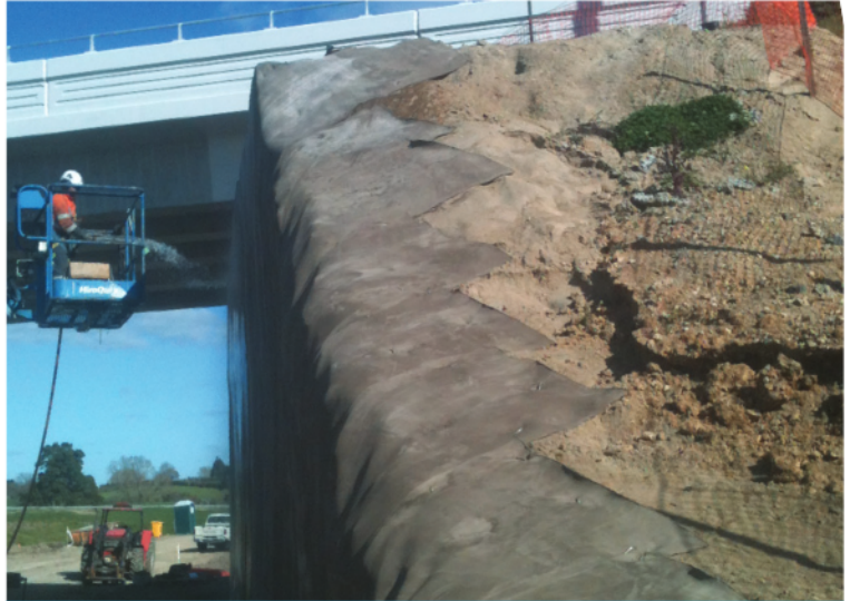
CC fixed in place with ground pegs and hydrated
