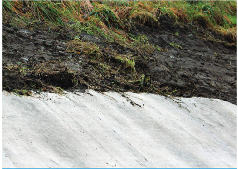
Anchor trenching of CC13 midway up the embankment.
