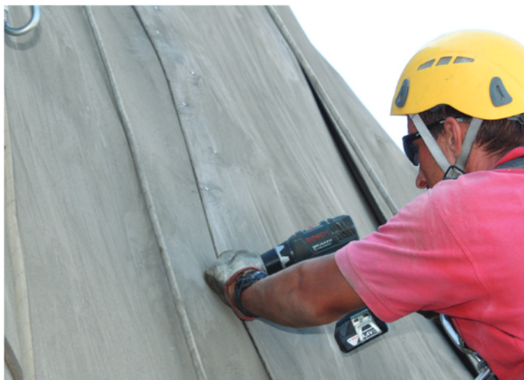
Every other screw was closer to the edge, forming a triangular shape
