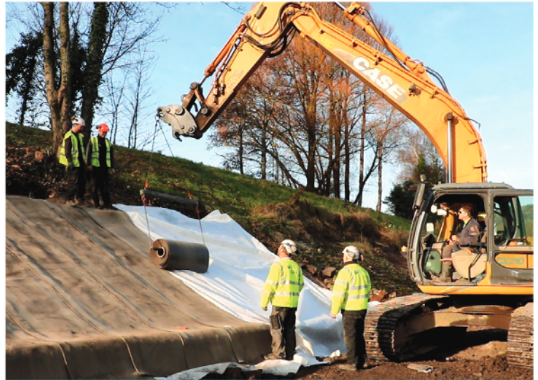
Deployment of CC over the geotextile
