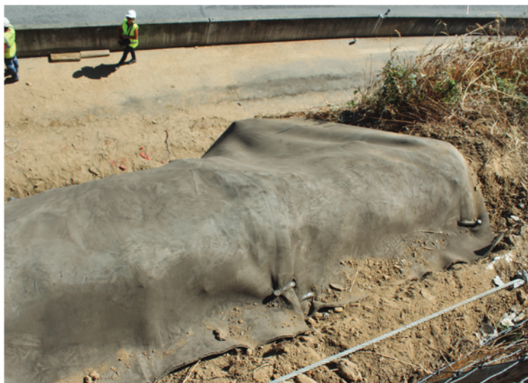
380mm ground pegs were inserted every 1m
