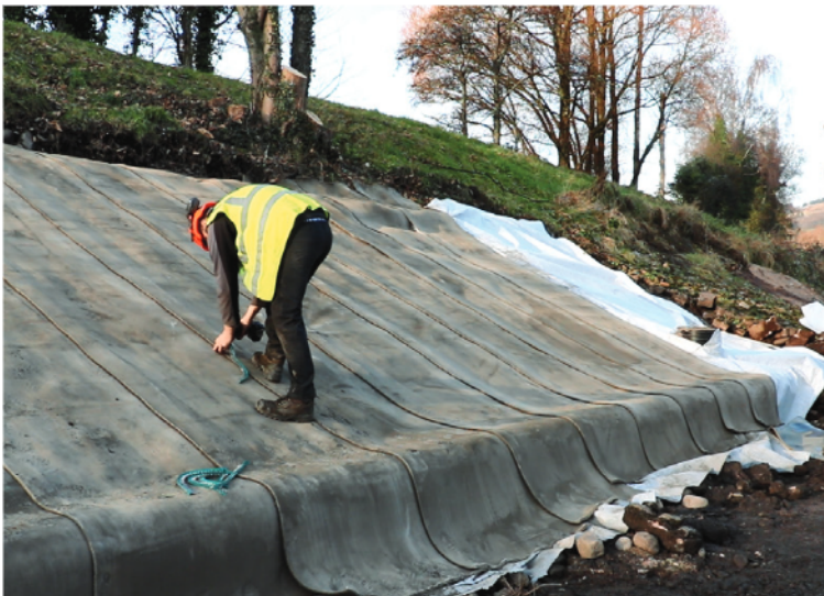
Fixing of the CC layers using screws
