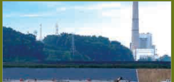
COAL ASH DISPOSAL
