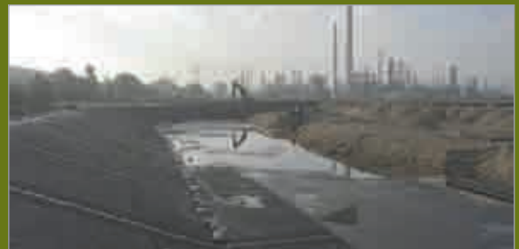
HAZARDOUS WASTE & CHEMICAL STORAGE
